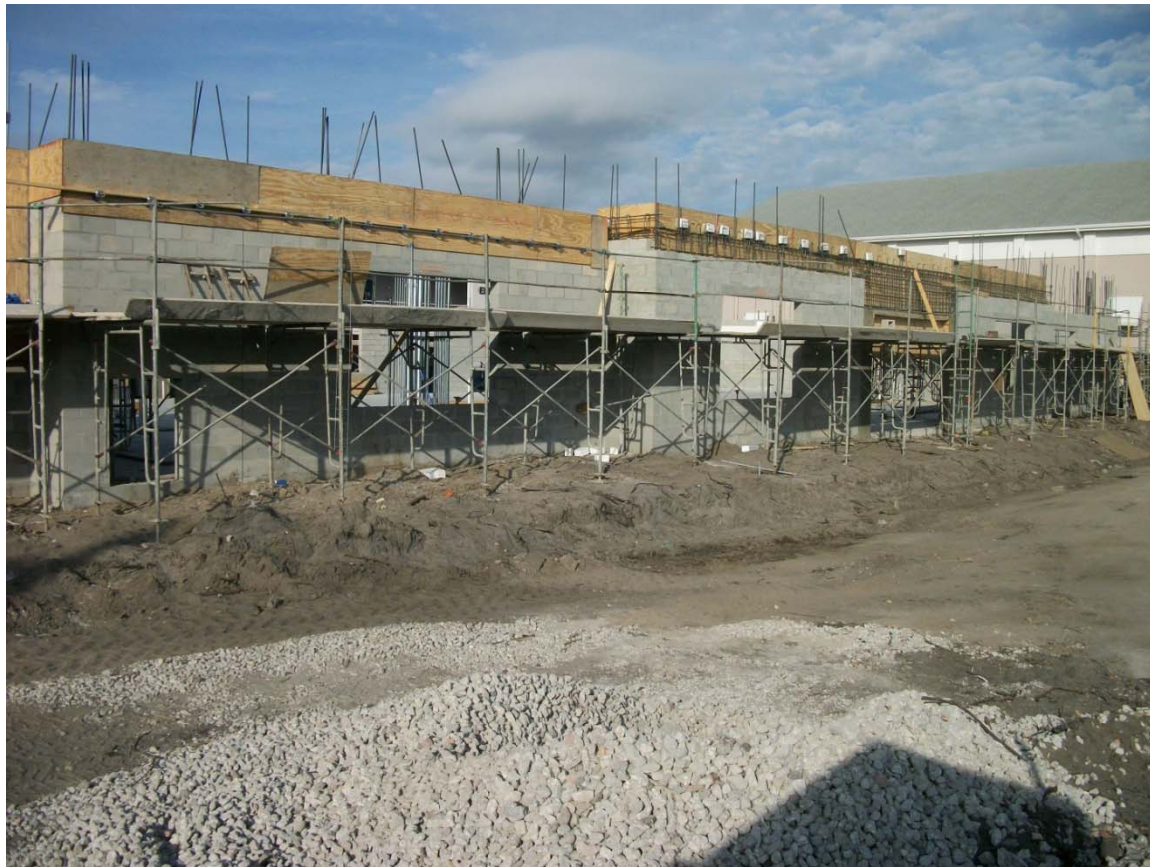
Top of wall tie beam construction in progress.
